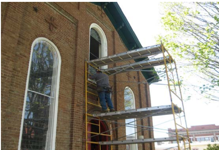
Stained glass windows being removed, piece by piece.
