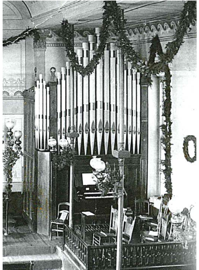
The old John Brown Organ - installed in 1898
