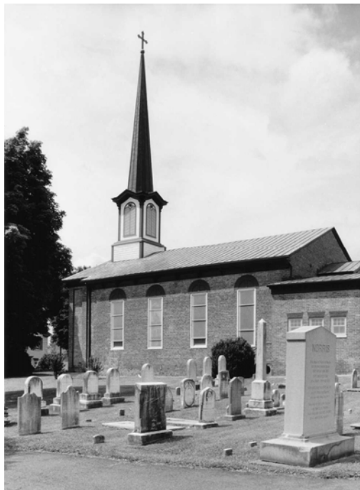
The cemetery is now located on the south side of the church.
