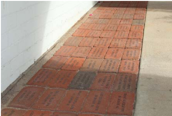
Memorial bricks are placed in the arch-covered walkway
